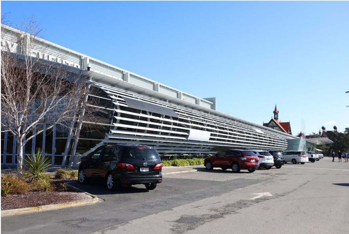
ATTACHMENT 1: FRONT LOOKING WEST BEFORE
