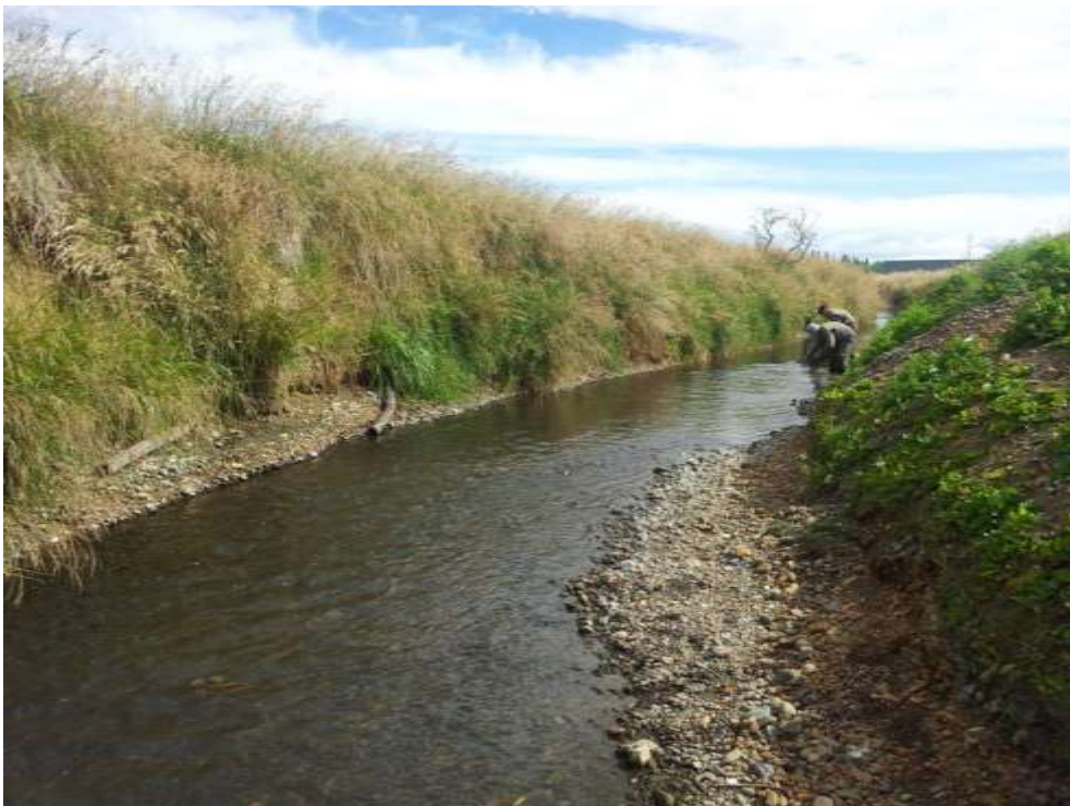
Photo 12: Another example of homogenous, post re-levelling habitat. Note the rapid, shallow flow on the outer bend. Exposed tile drain outflows can be seen on the left side of the picture.
