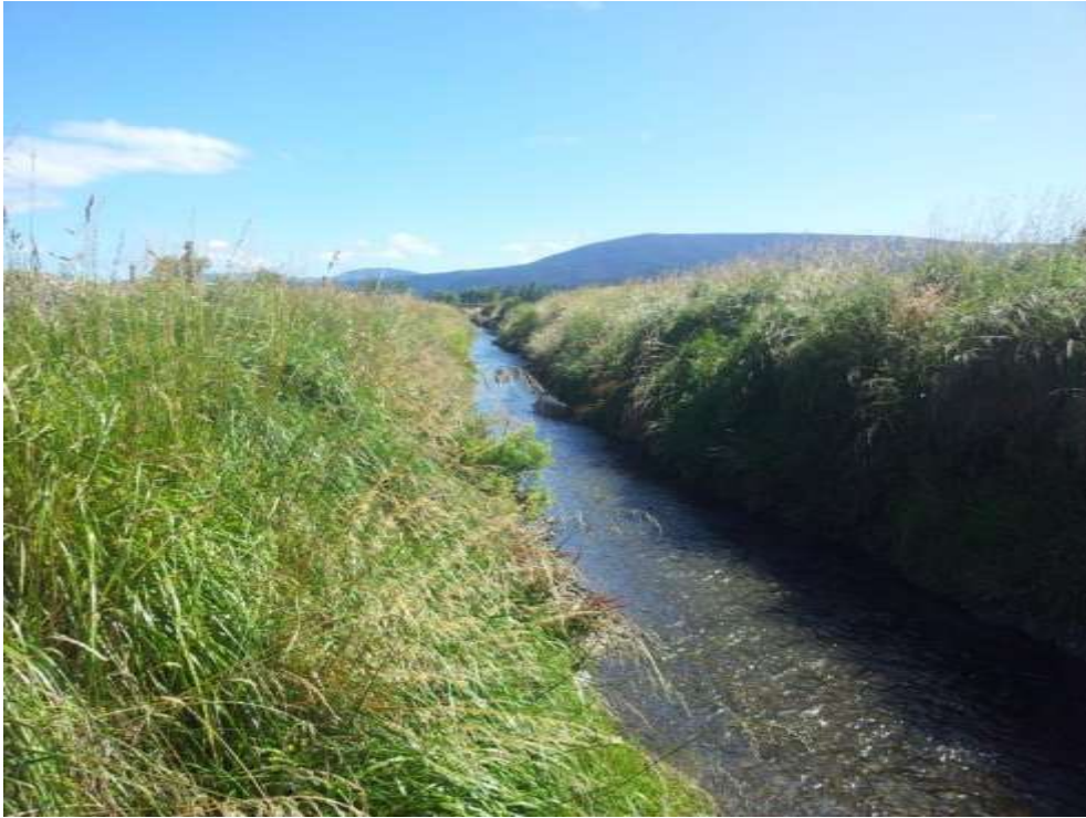
Photo 13: View from true left bank looking downstream towards the Longwoods forest. All large vegetation was removed as part of the re-leveling process.
