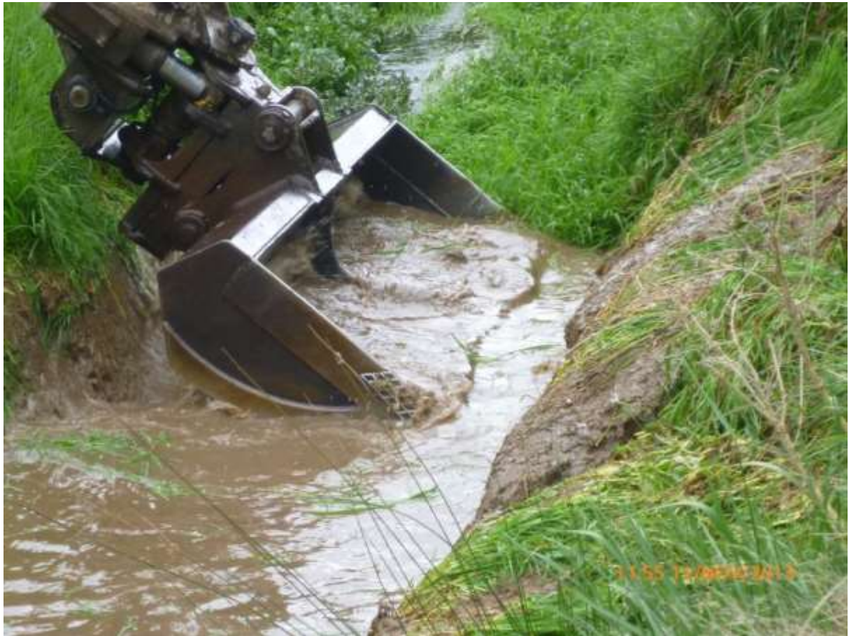
Figure 1: Typical mechanical clearance in Southland.
