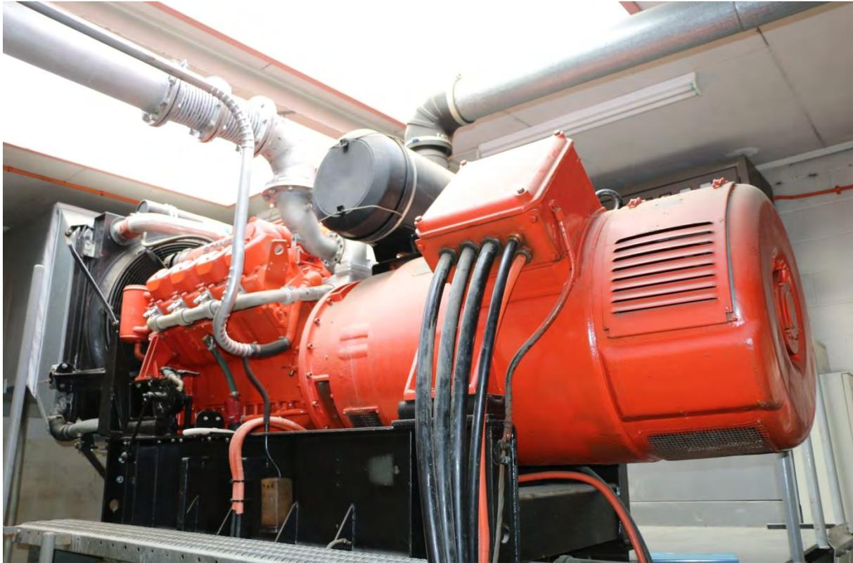
**Image 2: Standby Generator at Prestonville Pump Station, Waihōpai River**
