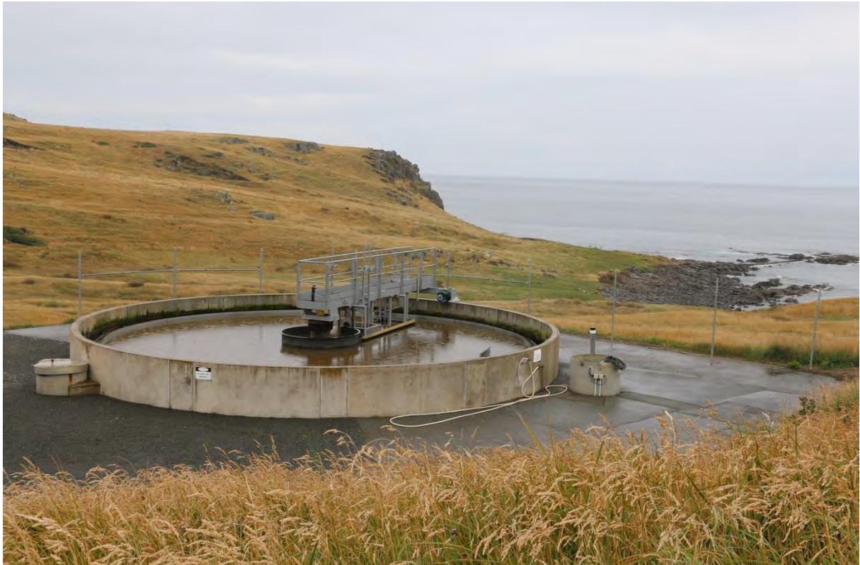
**Image C22: wastewater clarifier (the wastewater outflow pipe extends from the shoreline to the rocks on the right)**
