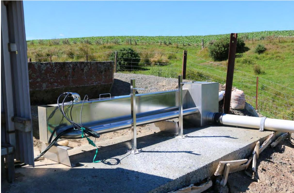
Image C9: Ohai ultraviolet disinfection reactor
