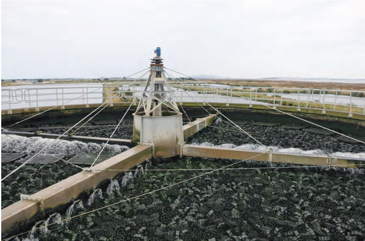
**Image C16: Clifton wastewater trickling filter**
