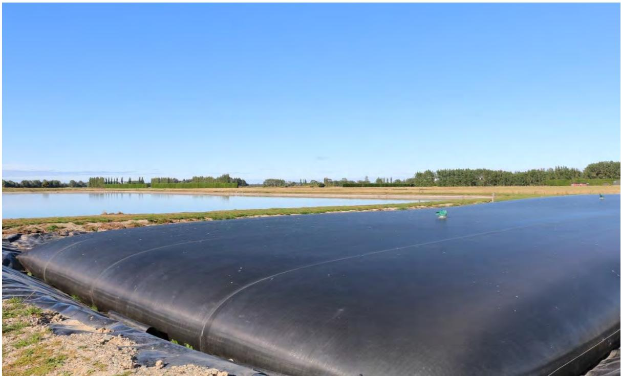
Image C6: Winton desludging geobag with oxidation pond in background
